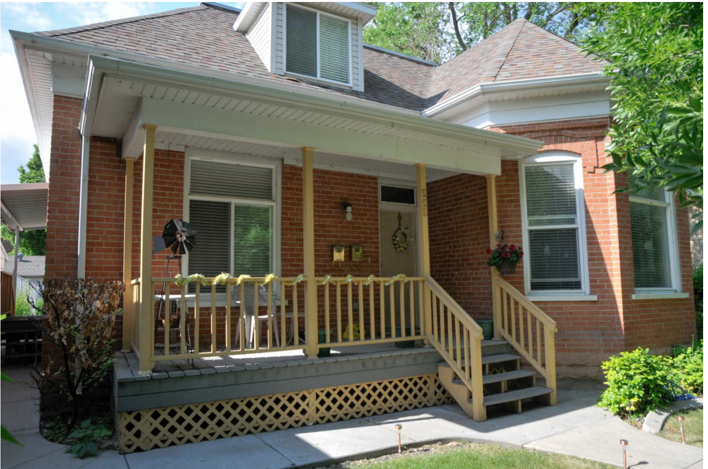
This single family residential structure is located west of the property in question at 555 West 400 North.
